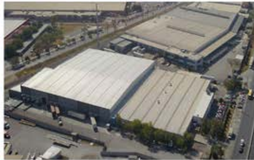
ACS Cleaning Products Manufacturing and Distribution Apodaca, Mexico
